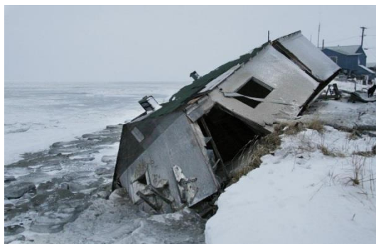
Figure 16 Melting permafrost and unusual storms are causing coastal erosion and property damage, including this house in Shishmaref, AK. Retrieved from http://motherboard.vice.com/read/climate-
