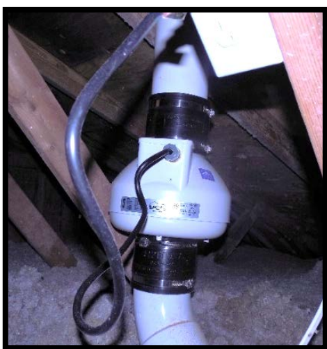
Active radon system with fan in attic.
