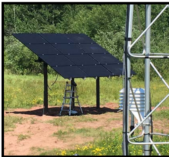
Installation of the 3.2kW solar array at Bad River's air monitoring site.
