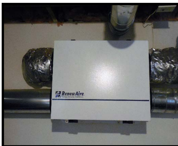
Heat Recovery Ventilator System.
