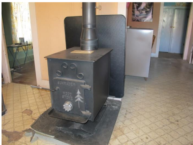
Forty year old stove vented through a masonry chimney that had never been cleaned. We had to close off and abandon the chimney, replace the hearth pad, and disconnect the trash burning in the kitchen.
