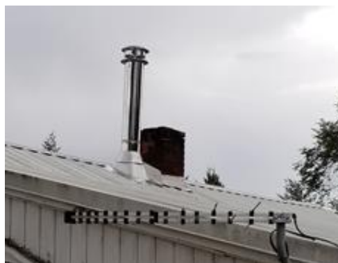
New Lopi Republic woodstove with new piping through the attic and roof.
