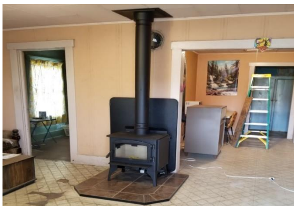
New Lopi Republic woodstove with new piping through the attic and roof.
