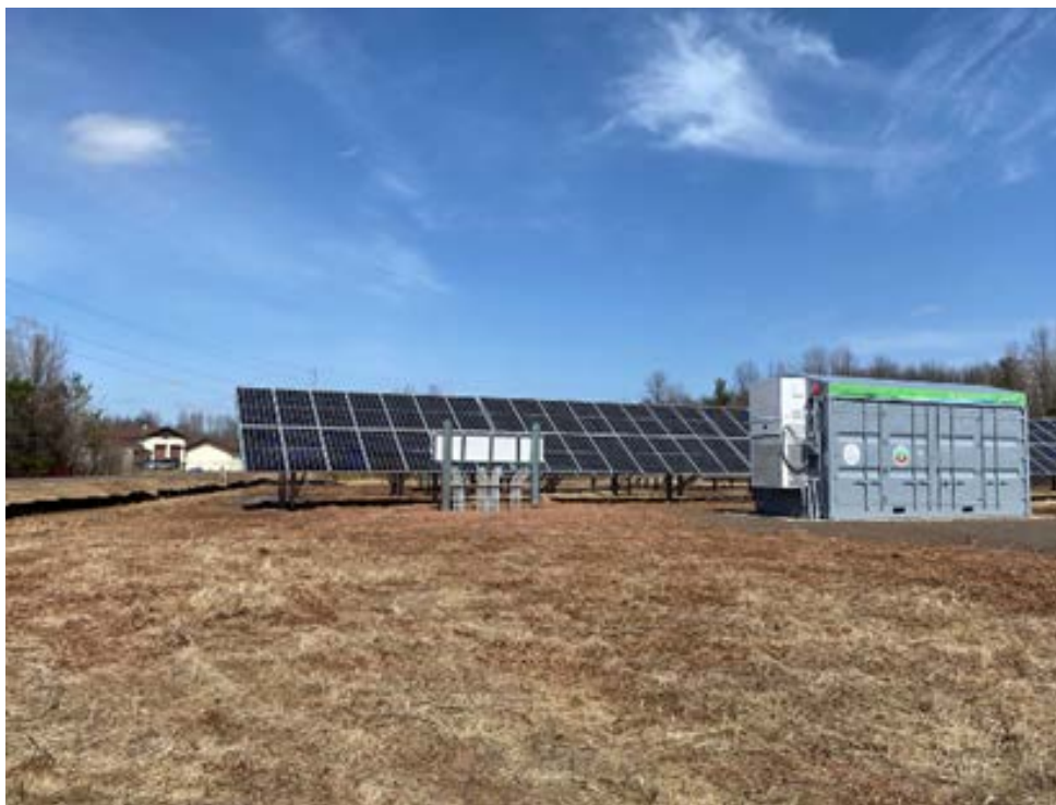
One of the three Tribal facilities, the new solar array installation, and the battery storage (gray metal box in the foreground) linking the array and the facility.
