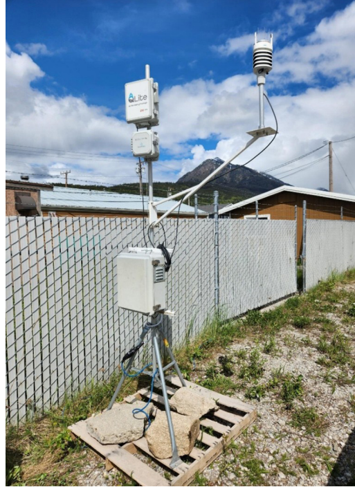
Figure 2: Water Department AQ Lite location
