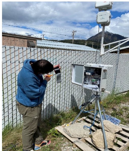
Figure 5: Colton Belisle repairing utility box component
